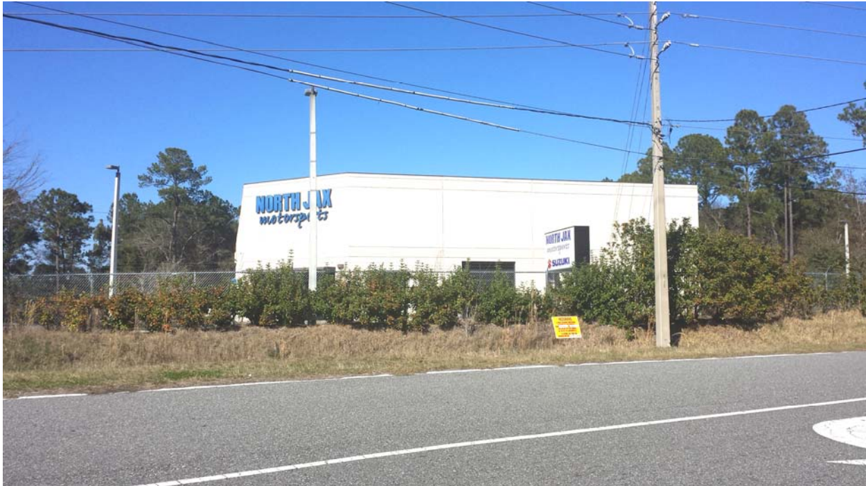
Figure 1. Subject property viewed looking north from Old Armsdale Road showing existing building and sign posted.
